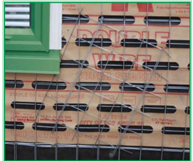
Sill with wire square reinforcement
