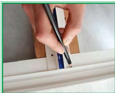
1. Measure the gap
