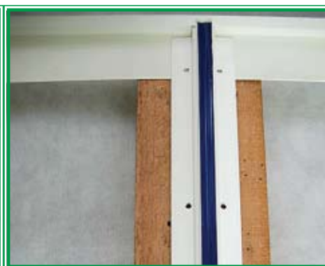
5. Attach at the top and along the length of the flashing
