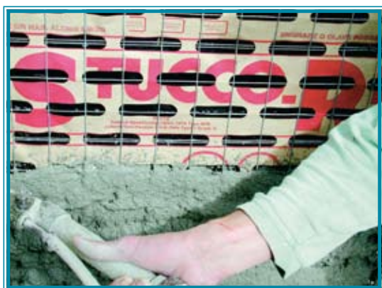
Fig. 1 Pumping Base Coat Plaster
