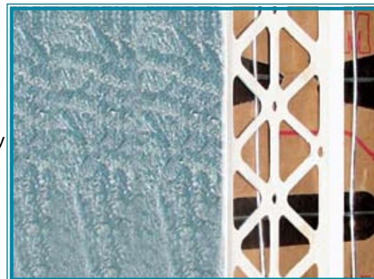
Fig. 3 Levelling and Mesh Coat on Corner
