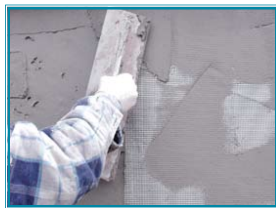
Fig. 4 Mesh Coat Application
