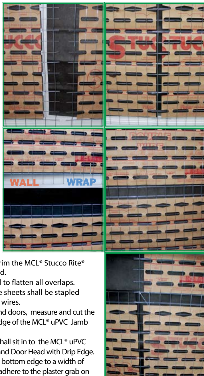
FIG. 1 Sheet overlap examples
