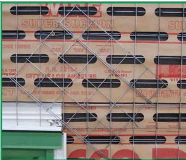
Head with wire square reinforcement
